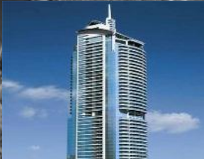
Movenpick Hotel, JLT 475 Rooms
