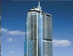
Movenpick Hotel, JLT 475 Rooms
